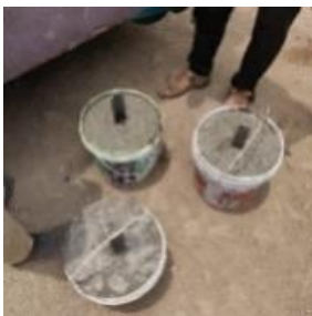
Figure 13: Bucket Foundation
